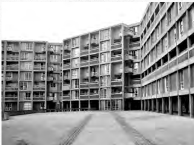
The Park Hill Estate, 1969. Photo's by Mick Jones
